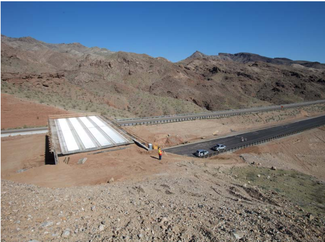
Figure 5. Sheep view of construction of sheep overpass at MP 12.2.
