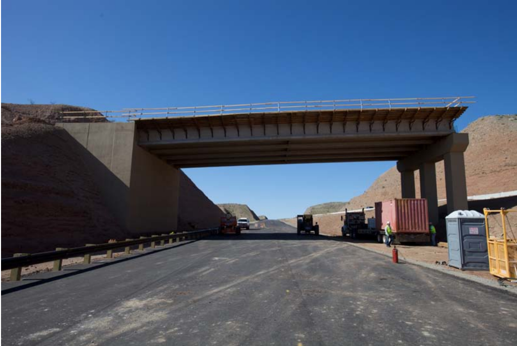
Figure 4. Side view of construction of sheep overpass at MP 12.2.
