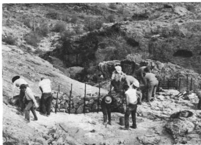
This diversion dam above Upper Mohave tank will protect the water hole from filling with silt and debris.
