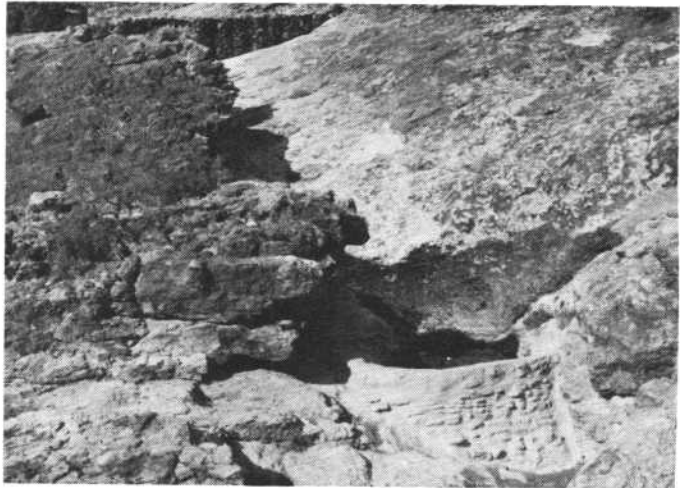
Upper Mohave tank — final results. The water tank is seen in the foreground, with the rip-rap diversion dam in the background.
