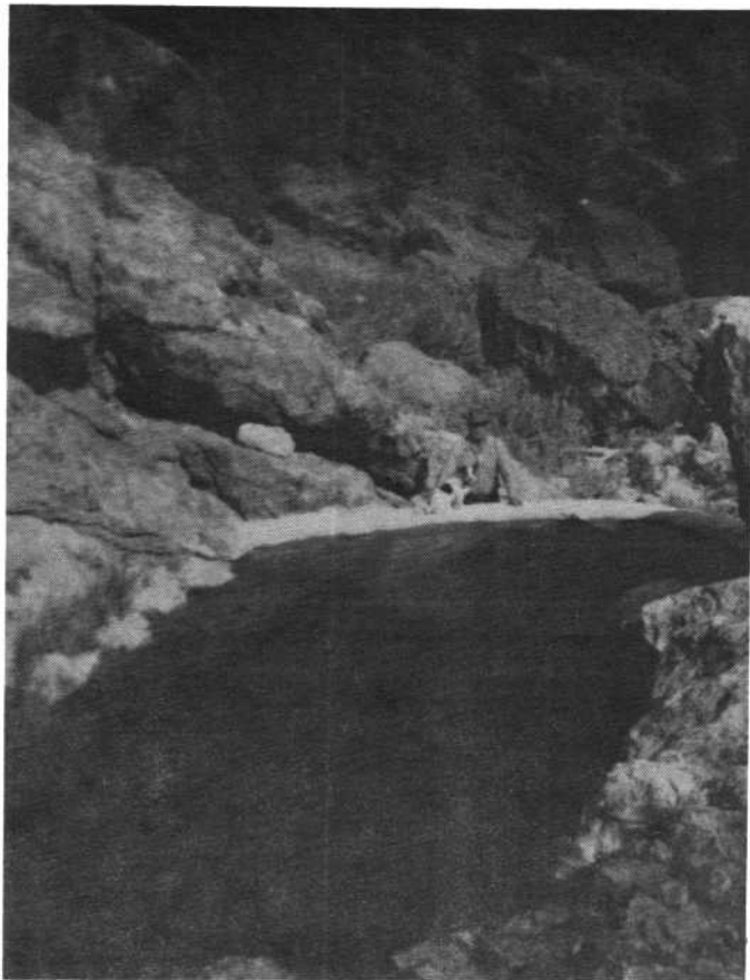
Upper Mojave Tank after renovation during the February 3 and 4 project by the Society. This photograph was taken by Carl and Anna Scrivens two weeks after a 1/2" rain. They reported seeing only three small seeps in the dam which is a great credit to all who participated in this memorable project.
