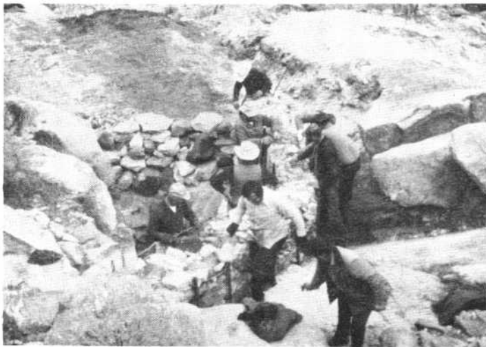
Rip-Rap Dam construction in progress.
