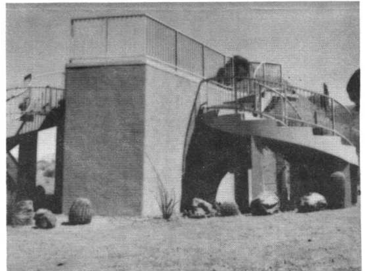
The completed Arizona Desert Bighorn Sheep Exhibit Building at the Phoenix Zoo.
