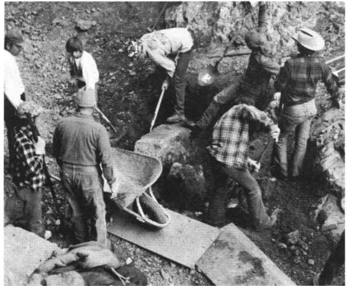
This scene shows the clean-up work in front of the Hidden Tank.
