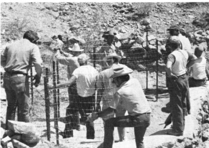
Erecting the wire mesh and supports for rip-rap dam.
