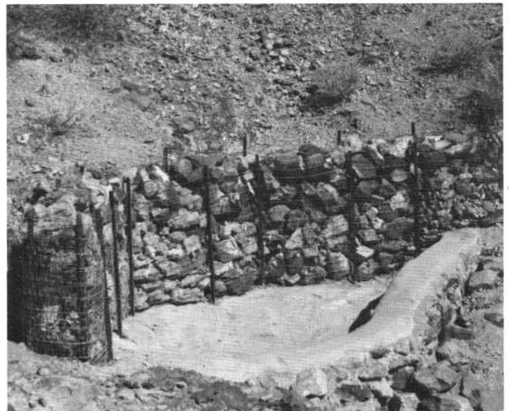
Little Horn Tank and its rip-rap retaining dam.
