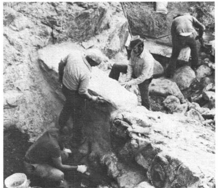
Joe Machac, Carl Scrivens and Cecil LeVance applying the final coat of Thoroseal to Lower dam.
