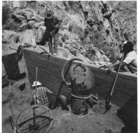
The "sand hog" that helped move an estimated 85 yards of fill in 1-1/2 days at Buckhorn Tank.
