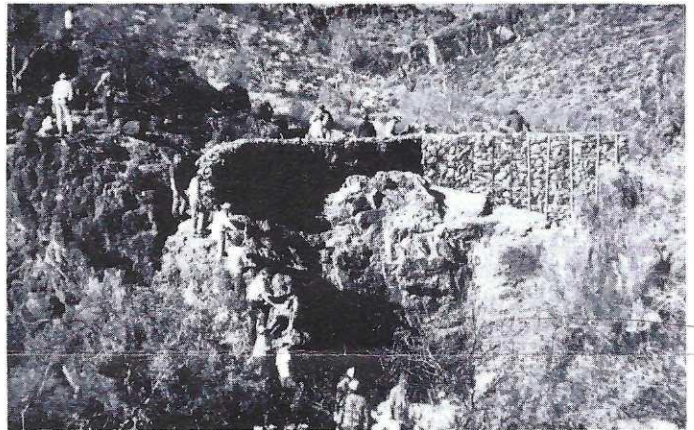
Completion of the Betty Lou Rip Rap Dam.
