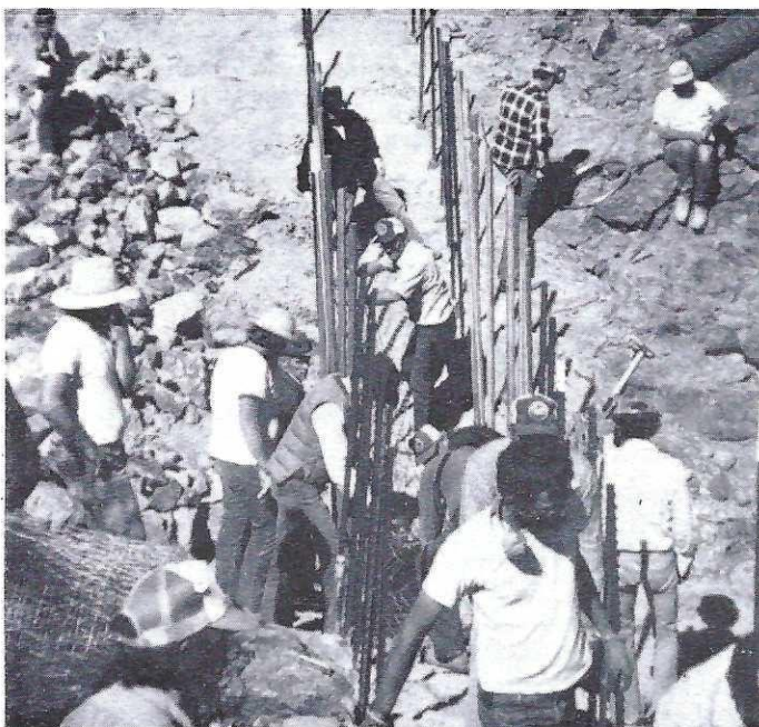
Construction of the Betty Lou Rip Rap Dam.
